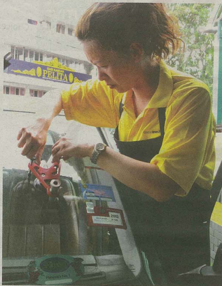
The injector has two functions, to extract air bubbles from the crack and to inject resin.
